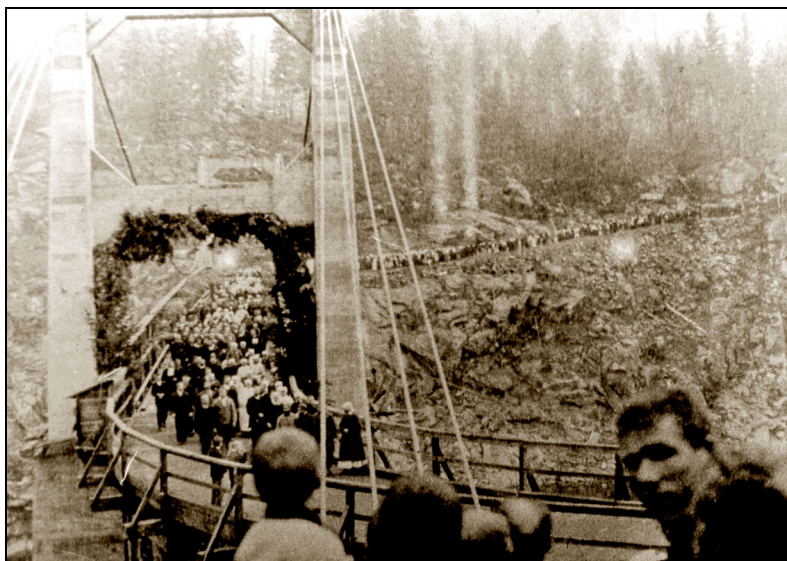
The opening of the Brilliant Suspension Bridge, October 1913 (from the Archives of the Doukhobor Village Museum, Castlegar, BC)
